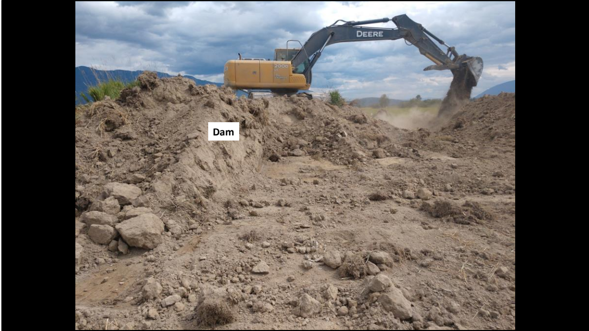
Here the excavator removes a center section of dam.
