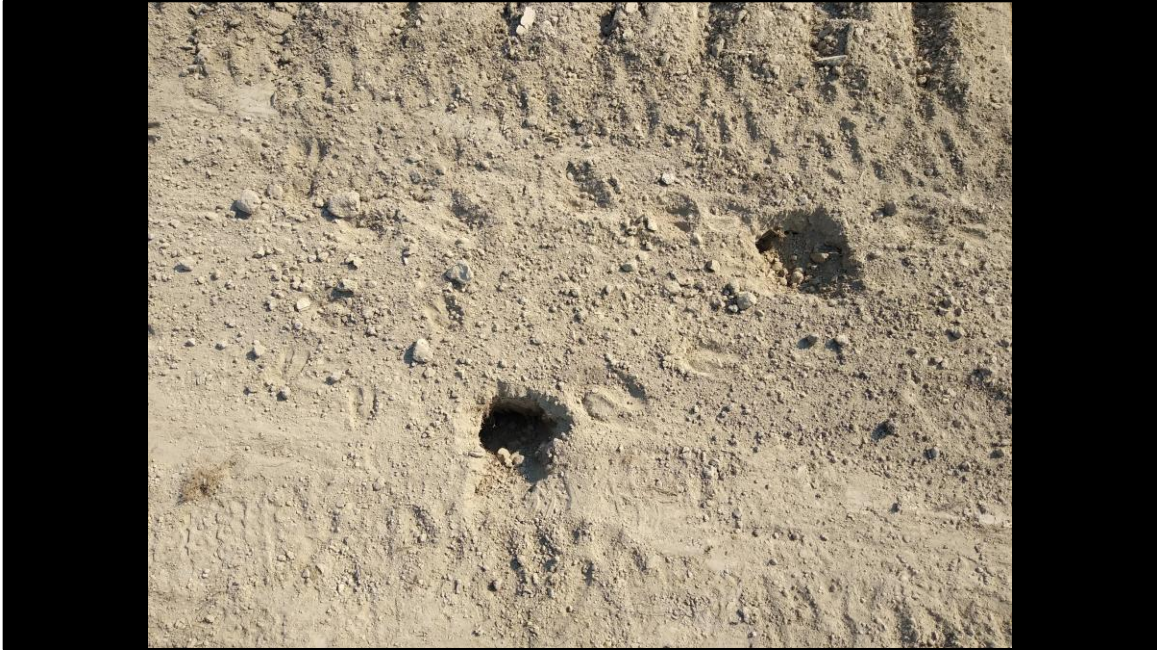
Here is a partially removed dam showing some of the many holes found in the dam.
