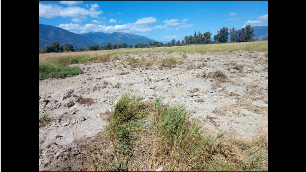
This photo shows another section of dam that was removed.
