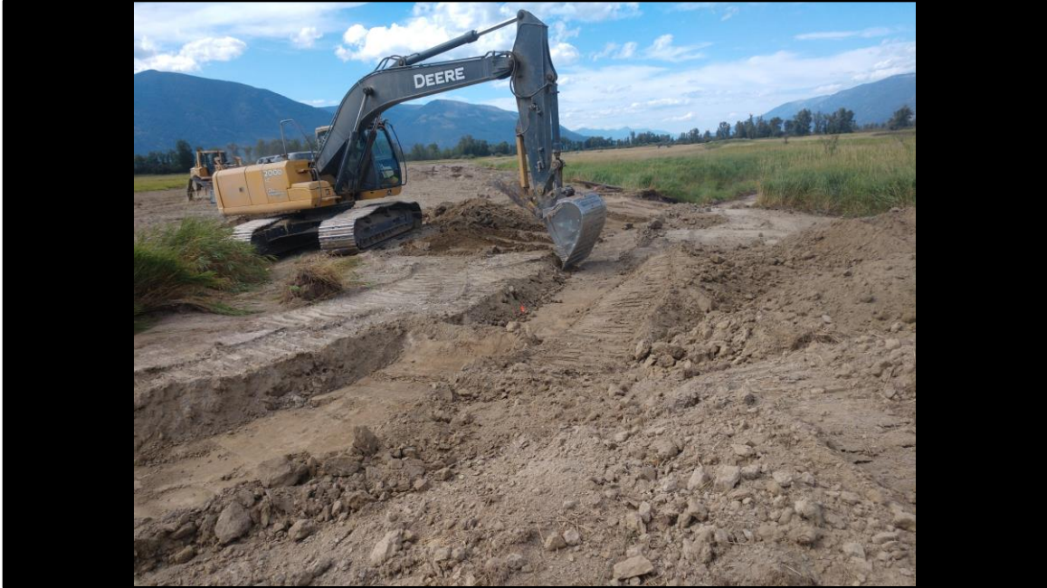
Gradual slopes are placed on the banks of the outlet.
