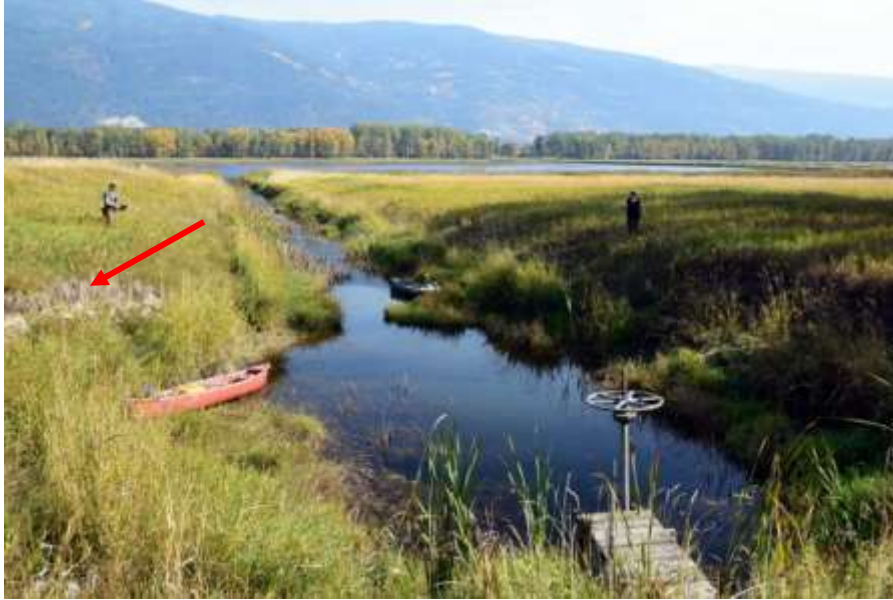
This is one of the channels dug to connect Six Mile Slough with the Kootenay River. Note the metal wheel on the water control structure, and an erosional head-cut shown by the red arrow.
