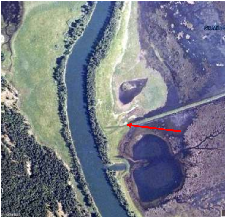
One can see where the natural peninsula was reshaped into the dike for wetland compartment 2 on this 2015 aerial photograph
