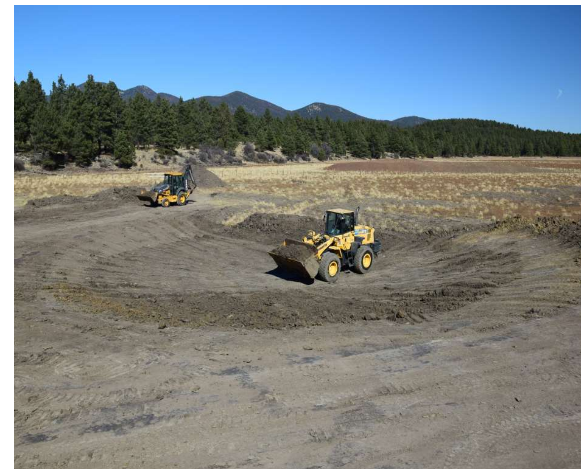
Figure 5. Compacting clay layers in wetland basin
