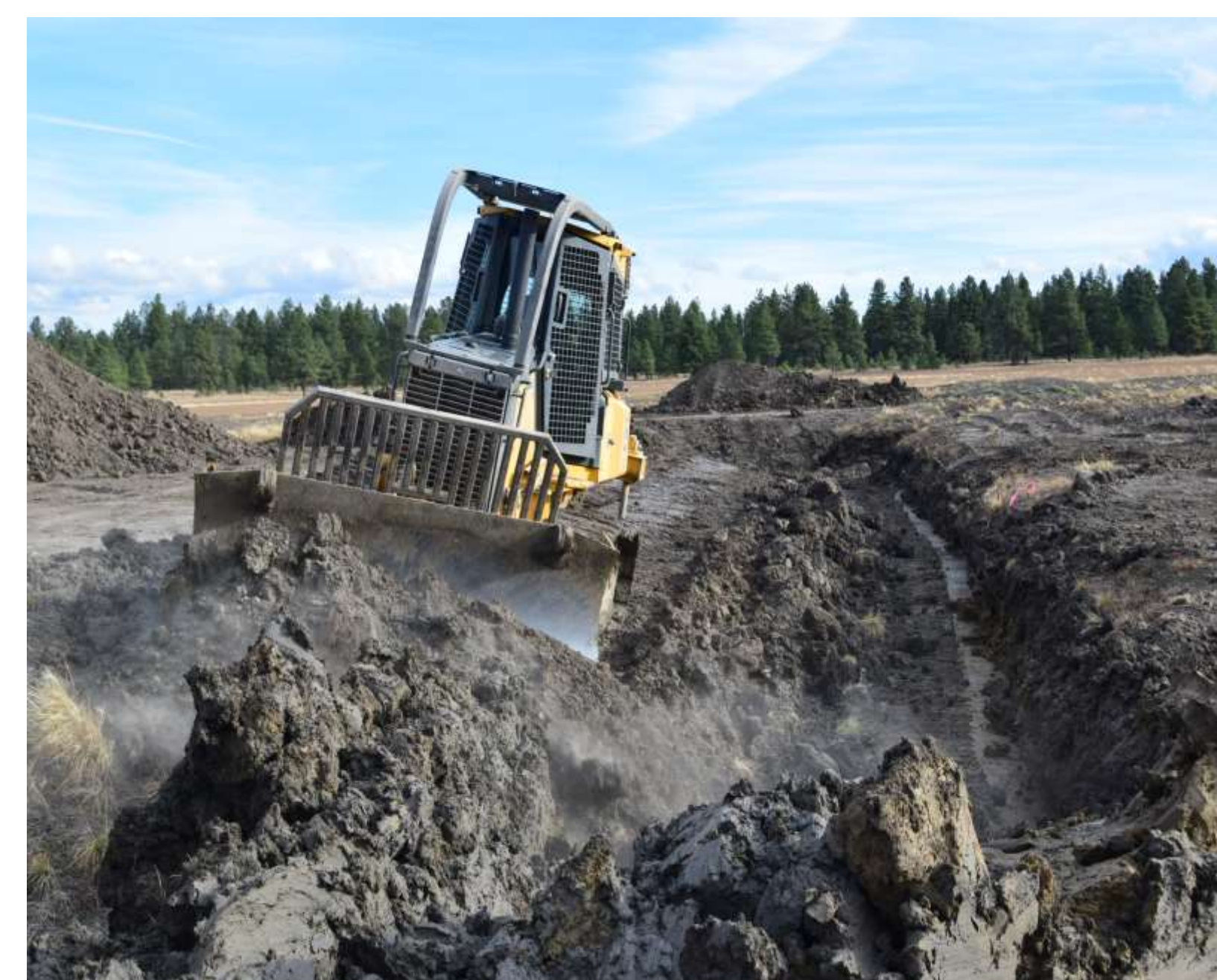
Figure 4. Reshaping ditches to obtain depth and slope
