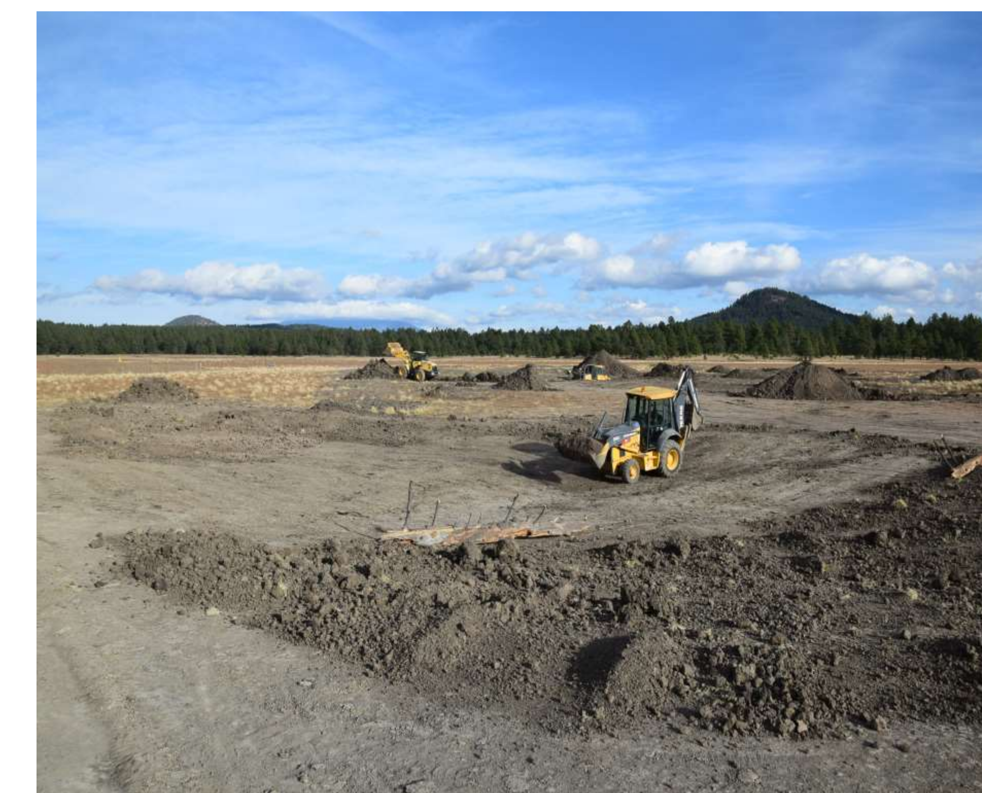
Figure 6. Spreading topsoil into compacted wetland basin
